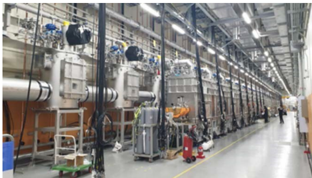
Figure 13: Installation work of HWR-B. Waiting for remaining 9 cryomodules.
