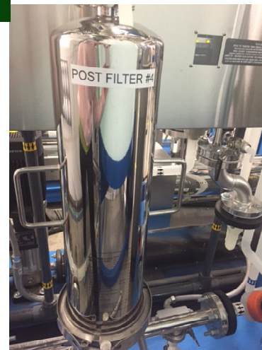
← Sub-micron post filter 0.02 \mu\text{m}
