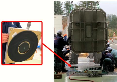
Figure 9: Installation of the air caster module.
