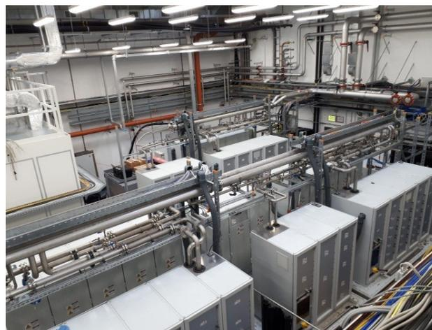
Figure 2: Klystron power supplies. Each power supply consists of two cabinets 32.6 kV 9.2 A, one combining cabinet and one rack for mains and controls.
