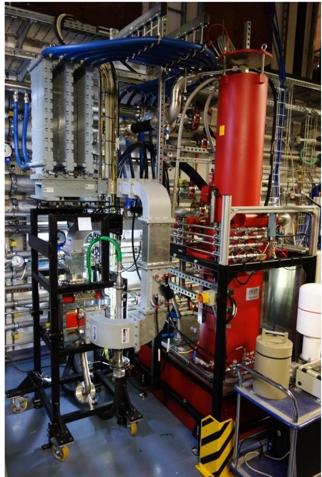
Figure 4: Installed klystron with circulator (left bottom) and 300 kW waterload (left top).
