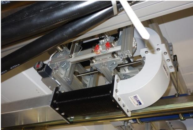
Figure 6: Motor actuated waveguide phase shifter.
