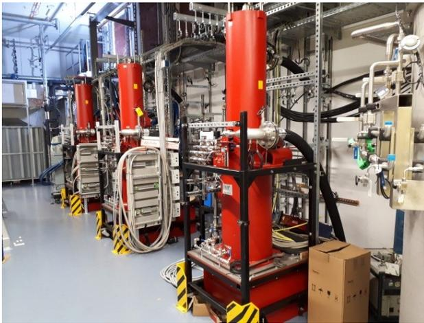
Figure 3: Installed klystrons.
