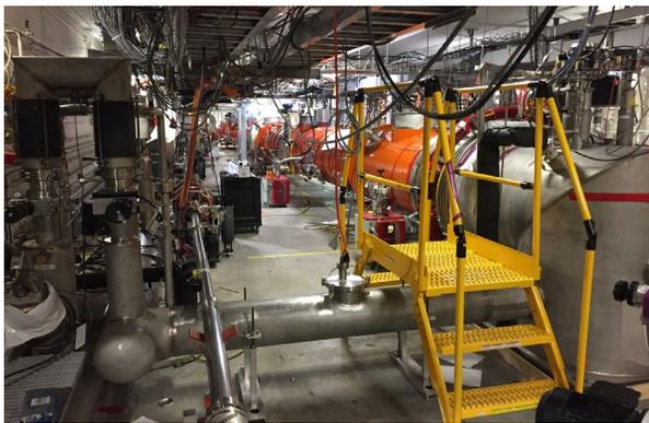
Figure 2: Showing the U tube, transfer line and cryo can connecting to the first cryomodule.
