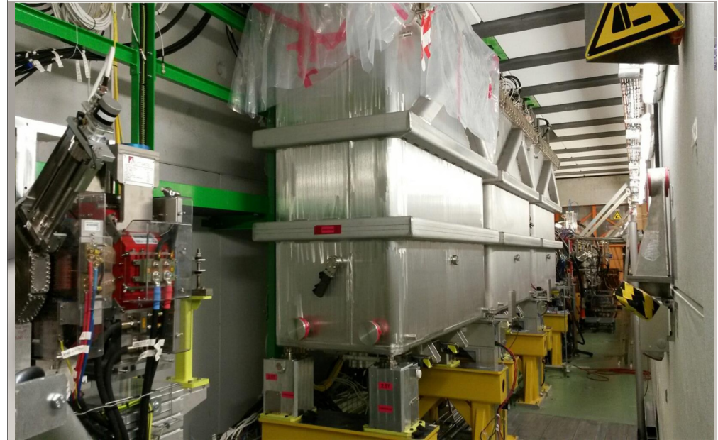
CM3 installed January 24 th
