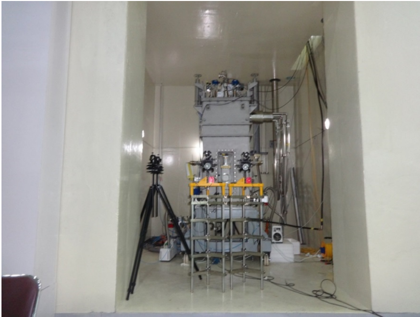
QWR Cryomodule (in test bunker)
