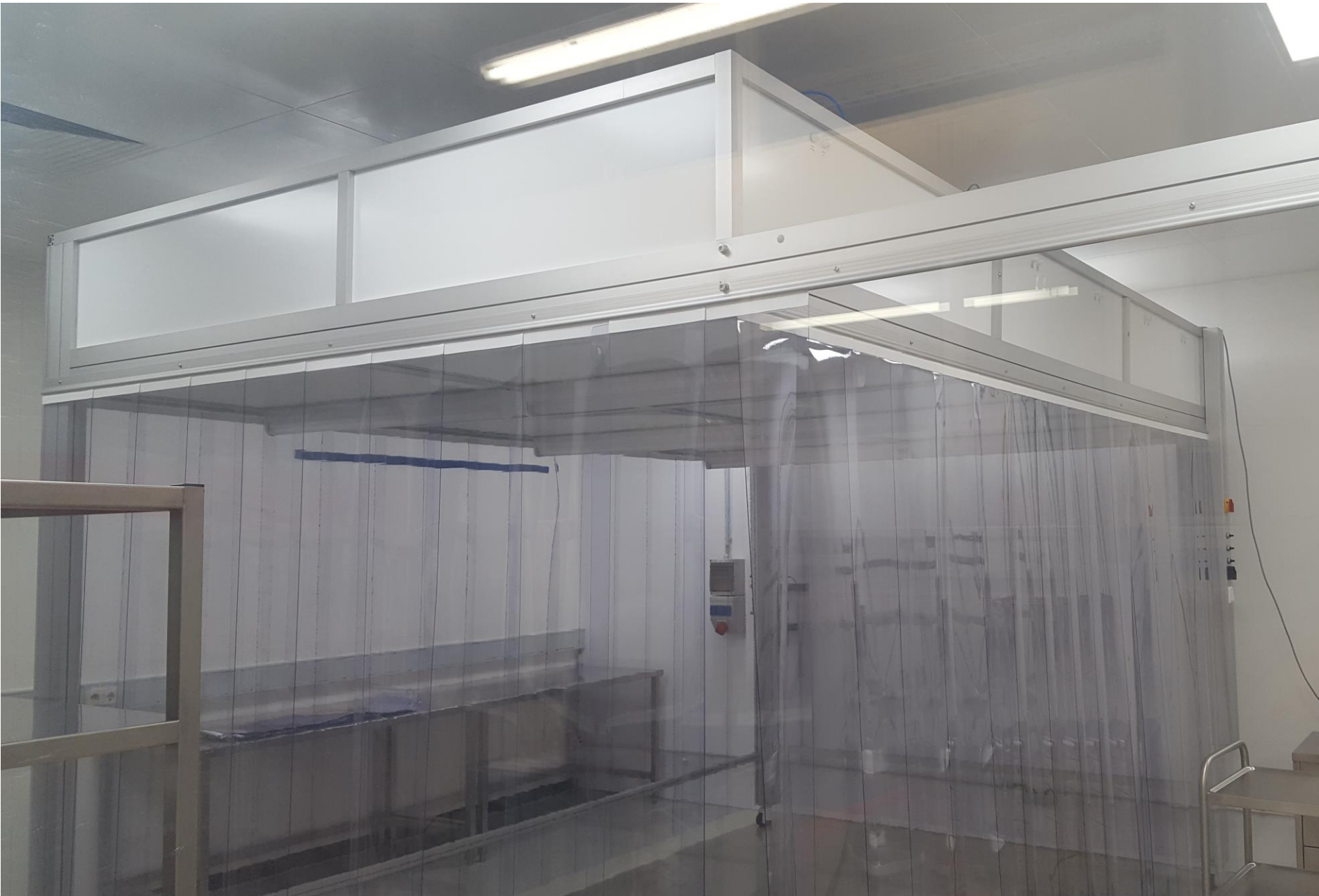
Cleanroom upgrade ISO 8 to ISO 4
