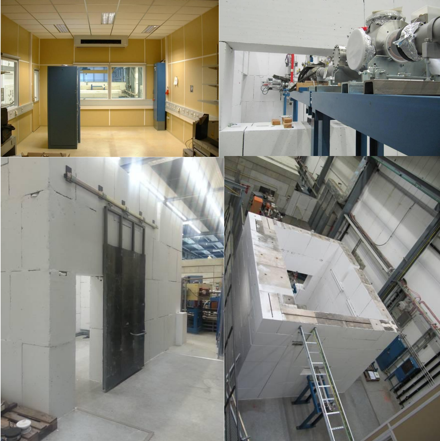
Protection cave for the cw-Demonstrator at GSI
