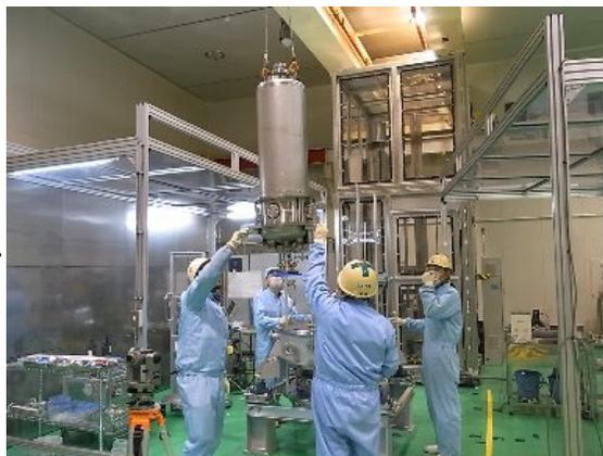
Figure 4: Heavy parts are brought into clean room using crane. Workers are wearing ISO7 clean ware and helmet.
