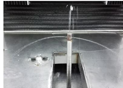
Figure 2: The nozzle of HPR system.
