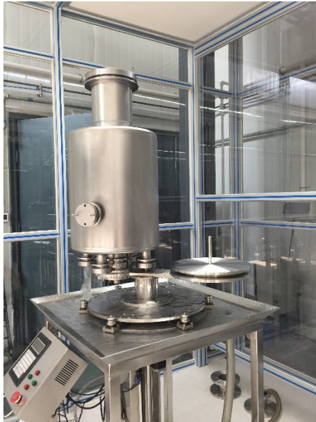
Figure 5: High pressure rinsing facility.
