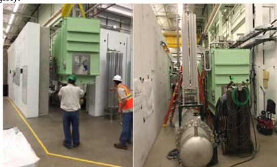
Figure 8: ReA6 bunker: during (left) and after (right) cryomodule installation.
