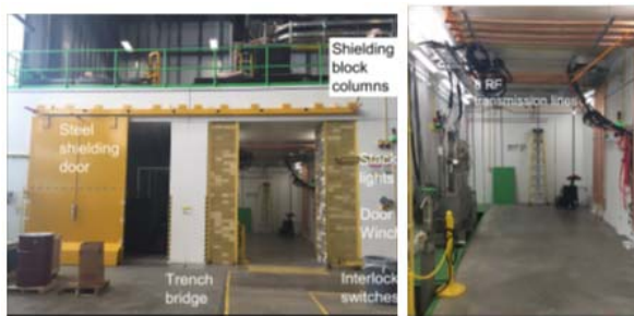
Figure 7: SRF High Bay bunker: exterior (left) and interior (right).
