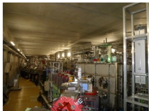
Figure 2: Injector cryomodule installed in beam line.
