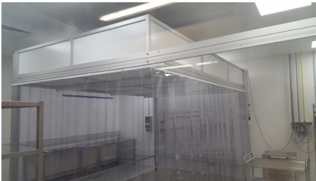
Figure 5: Upgraded cleanroom ISO 8 to ISO 4
