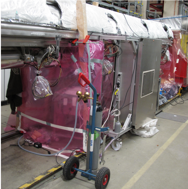
Figure 6: Local clean room at XM22 hanging at the cantilever for HOM antenna exchange.
