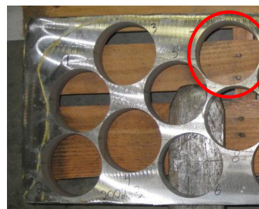
Figure 12: The bi-metal transition on helium vessel (Top) and the location cut from the leaked bi-metal transition (Bottom).
