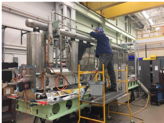
Figure 4: Pipe welding of the cryomodule inside.
