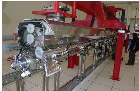
Figure 5: PXFEL2_2 cold mass hooked to the girder in the Roll-Out area.
