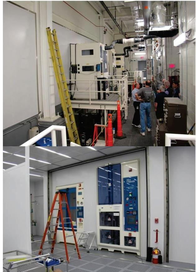
Figure 2: BCP and HPR tools bulk-headed into the new cleanroom and a view from the PSA.
