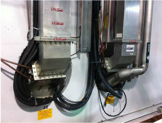
Figure 4: Typical CCL waveguide chases as viewed from the klystron gallery. The chase diameter is 0.61 m, and the waveguide size is WR1150.
