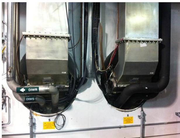
Figure 3: Typical DTL waveguide chases as viewed from the klystron gallery. The chase diameter is 0.91 m, and the waveguide size is WR2100.
