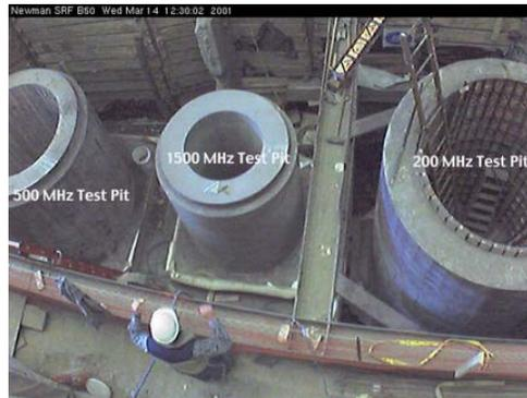
Figure 3: Test pits for various size cavities.
