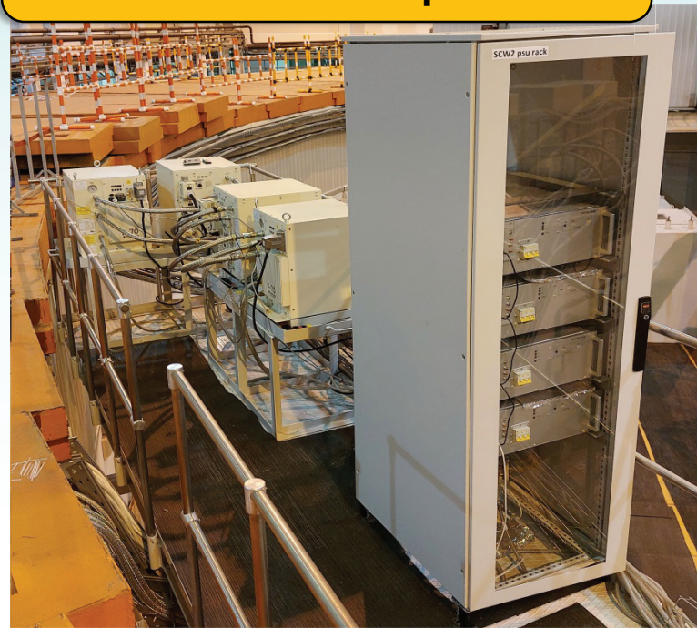
SCW power supplies, control rack & compressors
