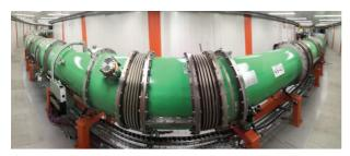
Figure 2: Booster ring in the tunnel inside the Synchrophasotron iron yoke.
