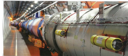
Beam-loss monitoring (BLM) chambers, two yellow tubes on the red secondary monitor on an LHC quadrupole magnet.
