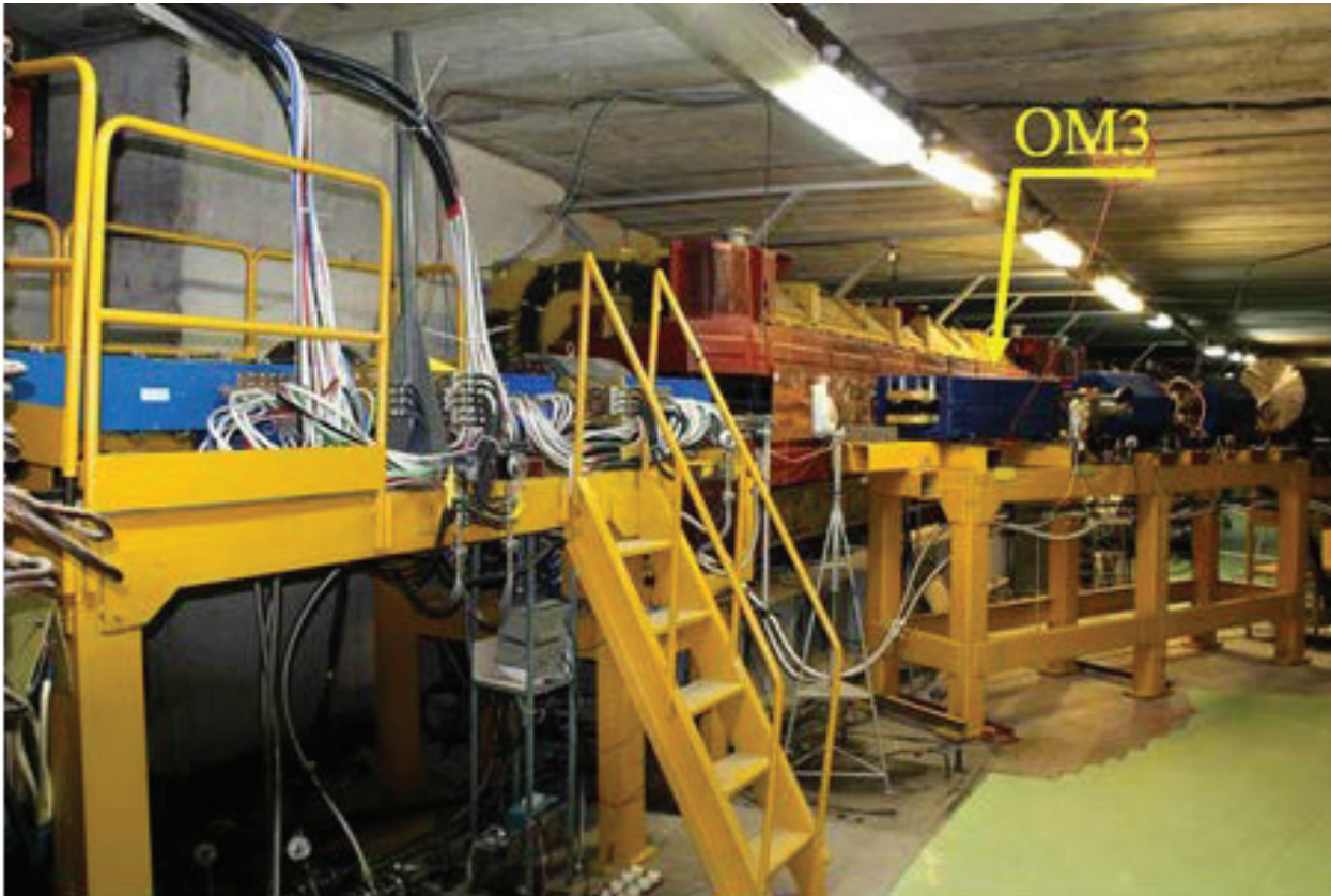
Initial part of transport channel
