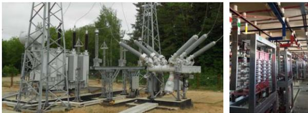
Figure 12: Direct connecting to an electric power transmission line 220 kV with a commercially available insulating gas (sulfur hexafluoride) electricity distribution switchgear (ABB) followed by a new step-down (10 kV) 108 ton transformer (left). Five sets of (static) thyristor AC-DC convertors designed and manufactured by the LLC “NIEFA–Energó” (St.-Petersburg) (right).
