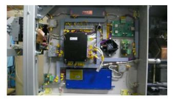
Figure 7: RF and cooling system controller.
