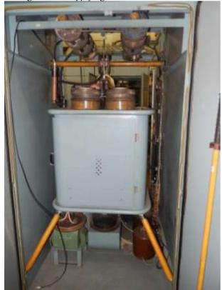
Figure 1: Modulator of the RF-generator.
