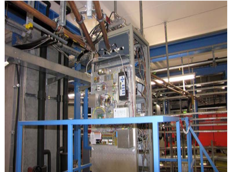
Test set-up of notch filter at ESR
