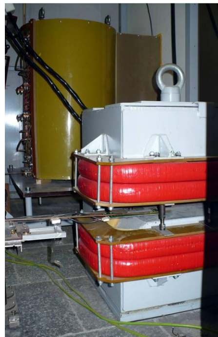
Figure 1: The kicker magnet at a test facility.
