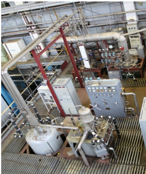
Figure 8: Cryogenic plant and large helium heat exchanger of superfluid refrigerator system of kaon channel.
