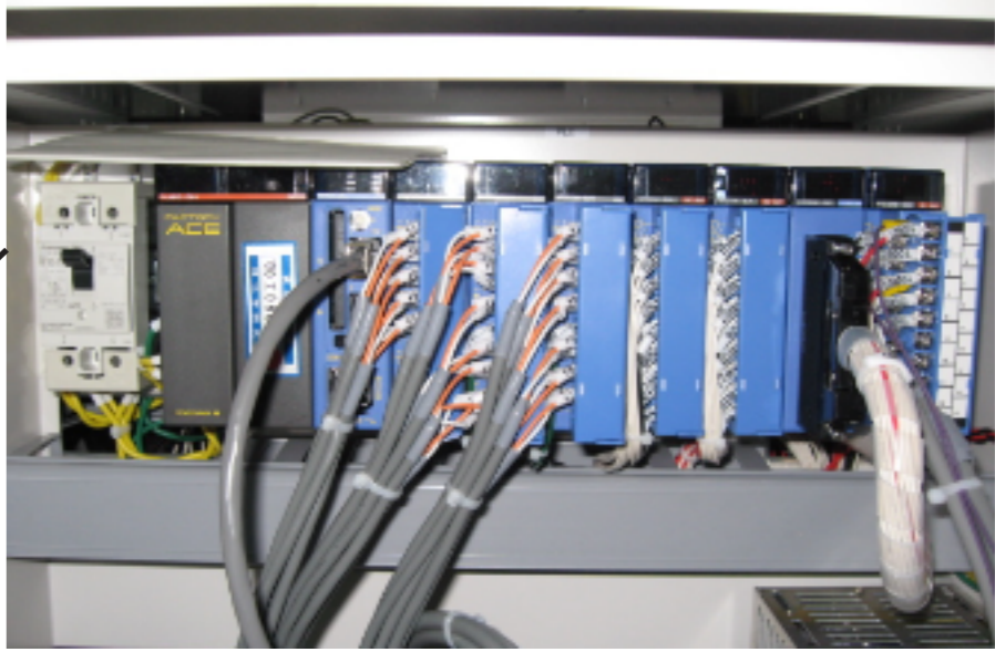
PLC-based system with Linux CPU. Implementation in 2009 for RIKEN 28GHz SCECRIS.
