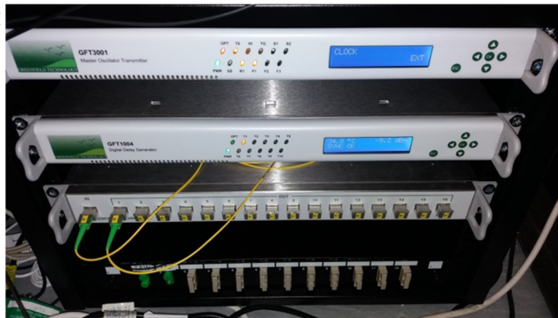
Figure 2: Installation of the GFT 3001 Master Oscillator and GFT 1004 Digital Delay Generator in Oscillator Room 2.
