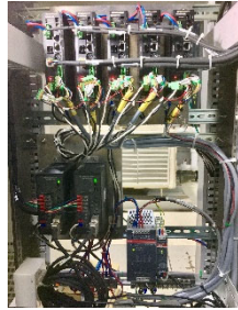
Figure 4: Installation of electronic drivers and controllers of stepper motors in a standard equipment rack.
