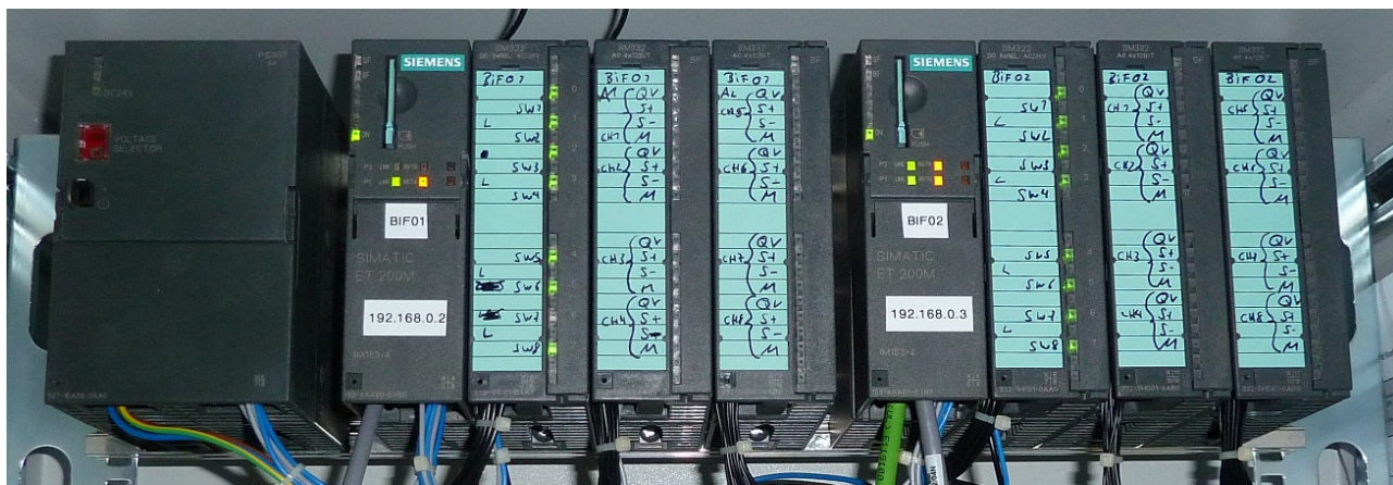
Figure 1: One of the 'satellites' of the BIF installation. It controls two BIF monitors and features two sets of control devices (from left to right): Power Supply, ET 200M controller, SM322 relay element with eight outlets, two SM332 12-bit DACs.
