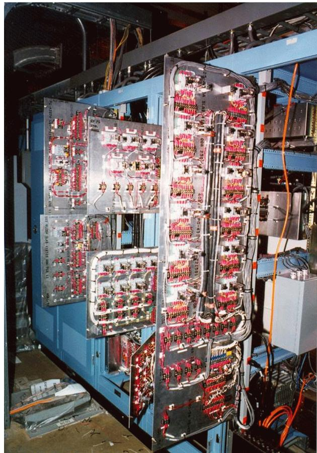
Figure 3: System interface relay panels.
