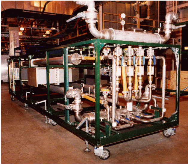
Figure 2: The rf load water system.
