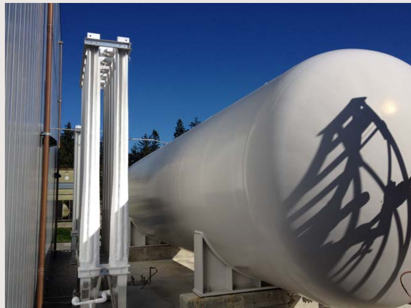
GHe storage tank leak-tested, evacuated and flushed with helium. Building an inventory for the compressors start-up. LN2 vaporizer is operational – sending flow of GN2 to dry carbon beds of ORS.
