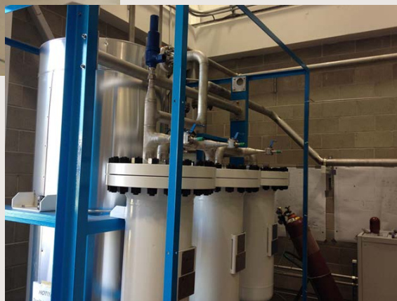
GHe storage tank leak-tested, evacuated and flushed with helium. Building an inventory for the compressors start-up. LN2 vaporizer is operational – sending flow of GN2 to dry carbon beds of ORS.
