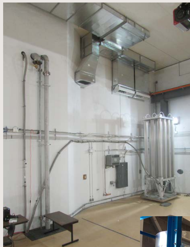
Warm He piping installed
