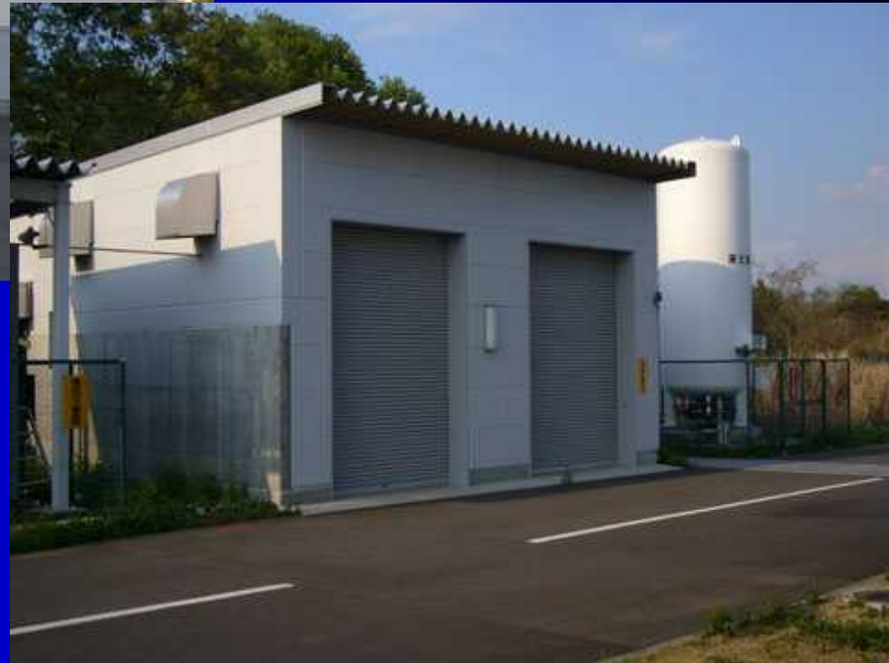
Compressor House and LN2 Storage
