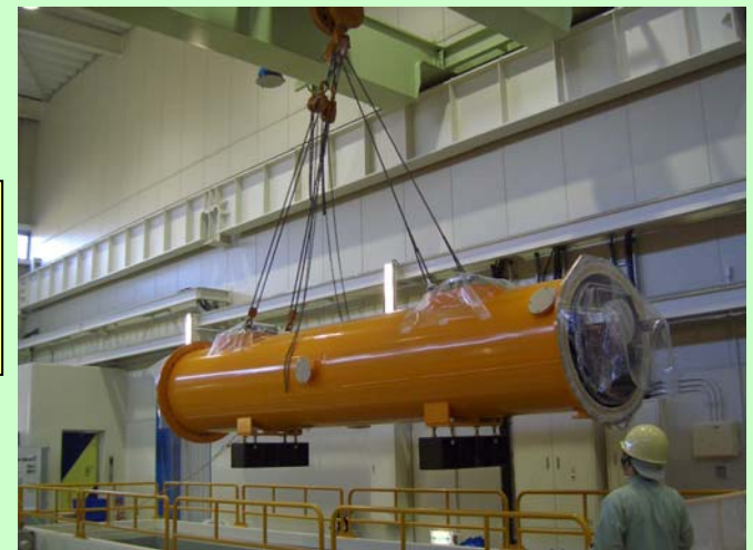
Vacuum vessel Assembly
