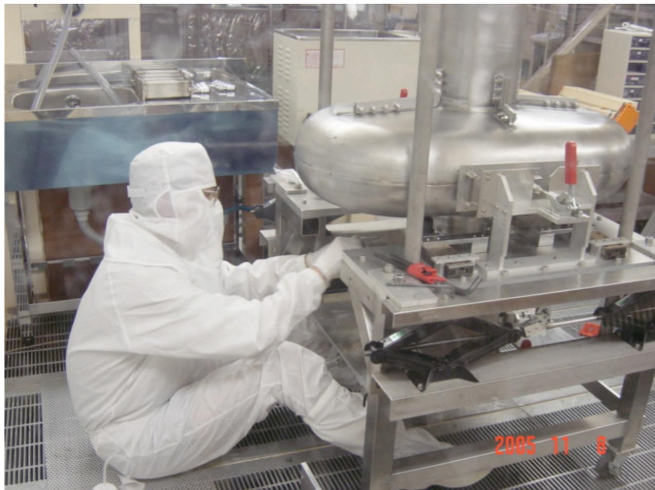
Set Flanges of Beam Pipes and Ports
