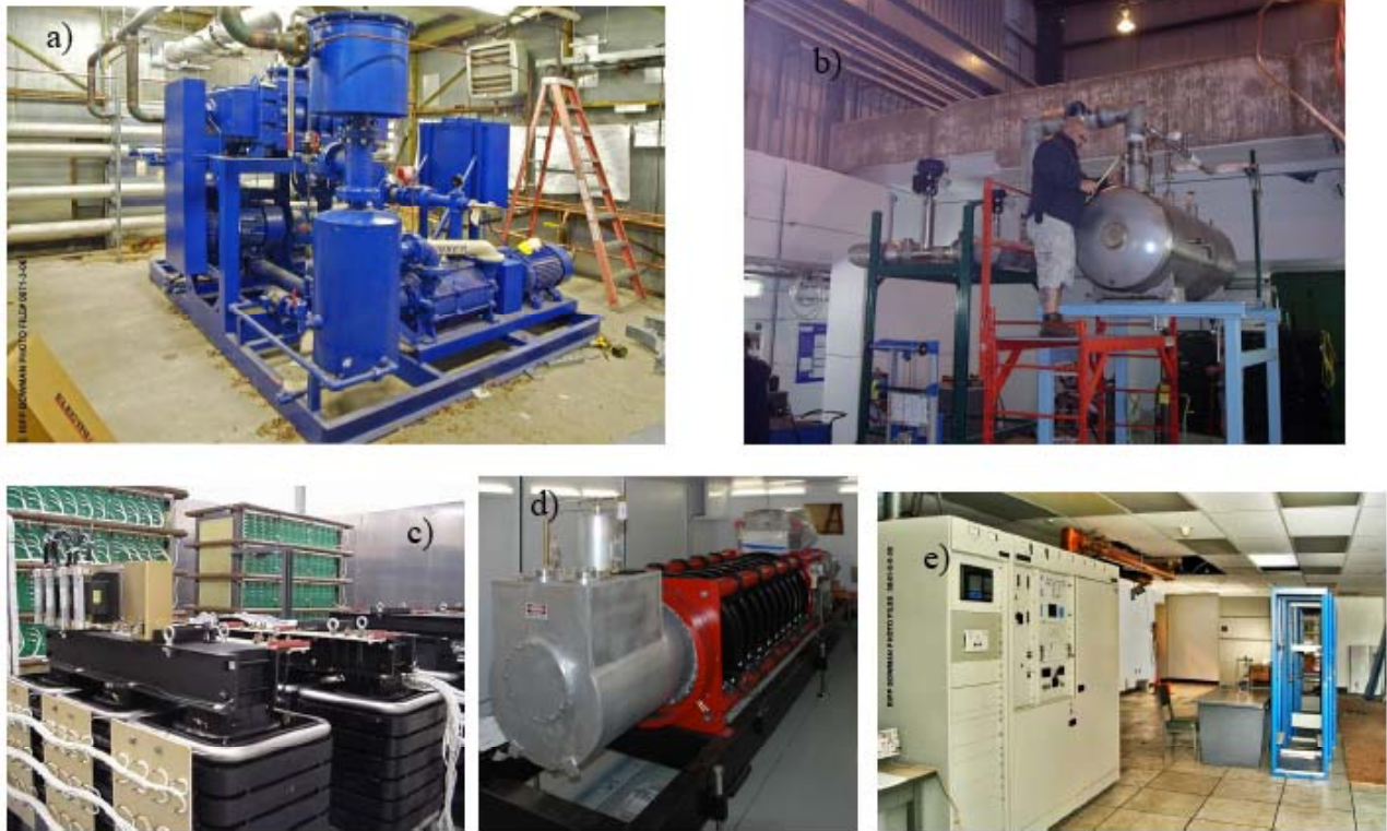
Figure 2: Some of R&D ERL subsystems: a) cryogenic pump for 1.8 K o operation; b) installation of ballast-tank for liquid He in the ERL shielded vault; c) 2 MW CW high voltage IGBT power supply installed in a dedicated air-conditioned room; d) 1 MW CW 703 MHz klystron installed into 2' steel garage; e) future diagnostics & control room with 50 KW 703.75 MHz transmitter and some racks
