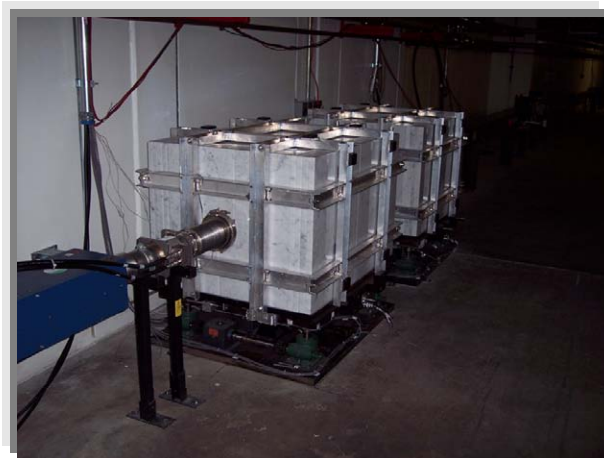
Figure 1: Collimators C836A and C836B with upstream magnet and bellows.
