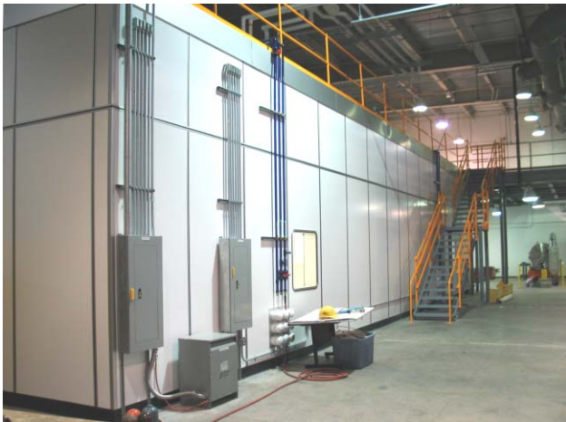
Figure 2: Exterior view of Cleanroom
