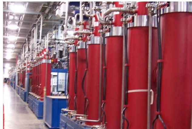
Figure 1: SCRF Klystron Gallery 550 kW klystrons
