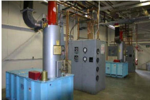
Figure 2: LANSCE klystron mounted in its modulator tank.
