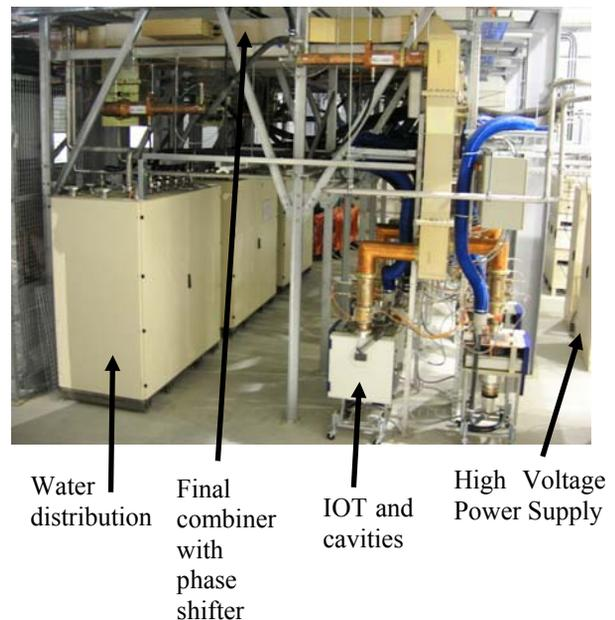
Figure 1: Photo of part of the RF installation showing IOTs with cavities, coaxial connection to waveguide combiner, the waveguide combiner running vertically up for the first combination and the horizontal section with phase shifter at the top of the picture.
