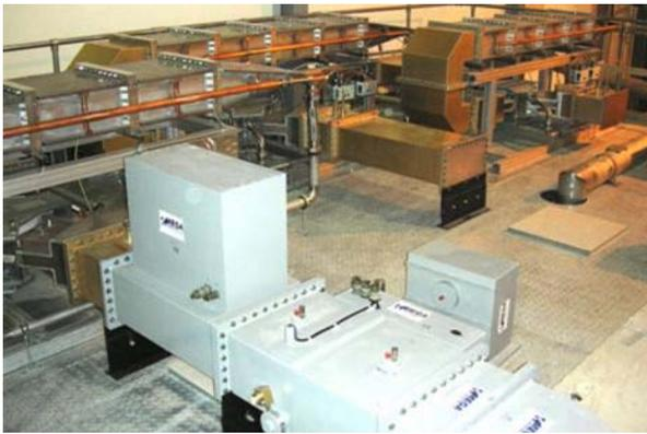
Figure 2: Photo of the high power circulator with 300 kW ferrite loads wrapped around the top. In the foreground the three stub tuner and the waveguide switch are visible.
