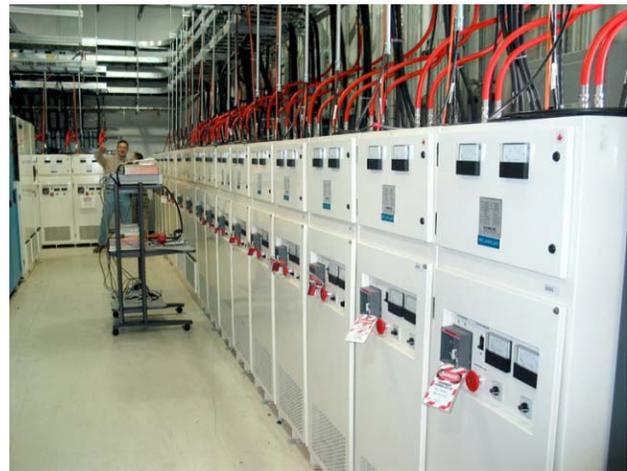
Figure 4: HEBT Quadrupole and Dipole power supplies.
