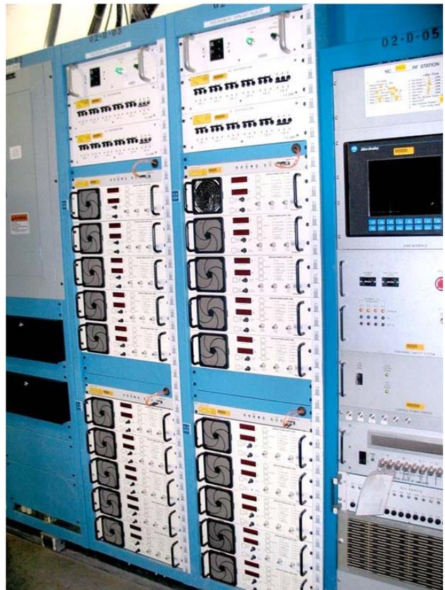
Figure 1: Four of the DTL dipole magnet corrector power supplies, Master-Slaved to +/- 100 amps.
