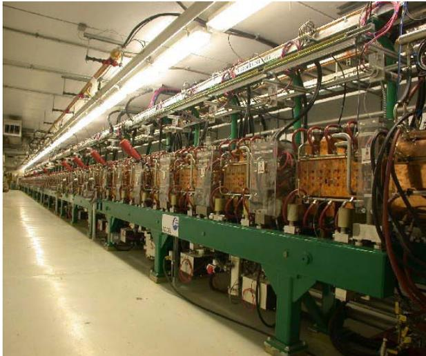
Figure 3: Completely installed four CCL modules in the linac tunnel.
