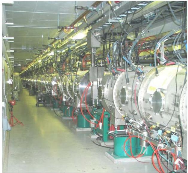
Figure 4: Medium beta cryomodules installed and ready for RF testing.
