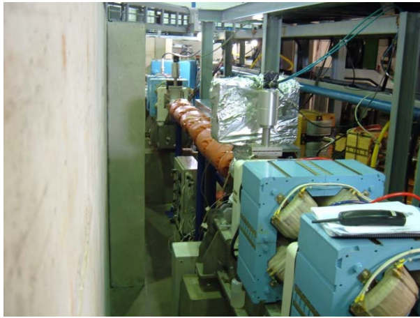
Fig. 3 NEG activation of the wiggler chamber during installation
