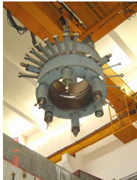
Figure 2: Cryostat assembly during installation.
