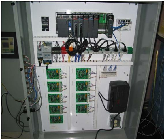
Figure 2: Electronics Base and PLC Controller.
